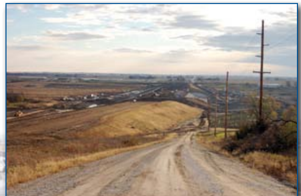
The Lake Wanahoo dam site, looking east along the former County Road M in November 2009.
